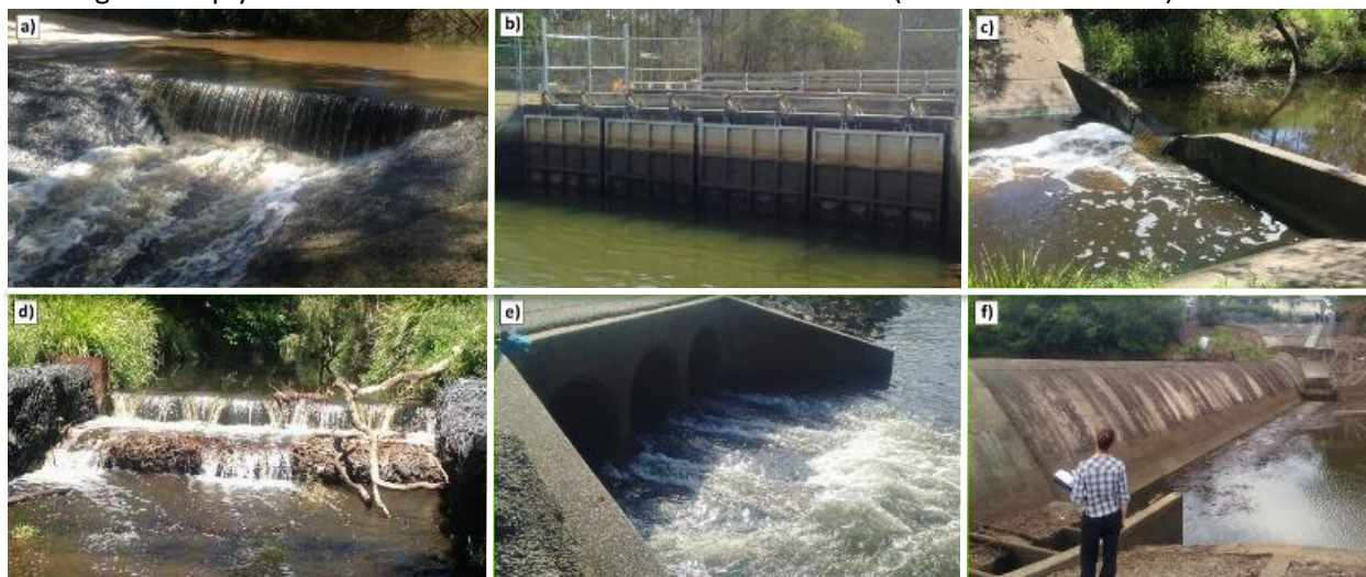
Figure 2. Barrier structures: a) Road causeway & concrete apron (Elimbah Creek), b) tidal floodgates (Behm Creek), c) V-notch stream gauging weir (Warrill Creek), d) Sheet pile and gabion basket weir (Warrill Creek), e) pipe culvert causeway (Albert River) and f) Tidal barrage (Caboolture River).
