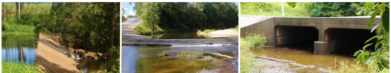
Figure 5. Left to right: low passability barrier, medium passability barrier, high passability barrier.
