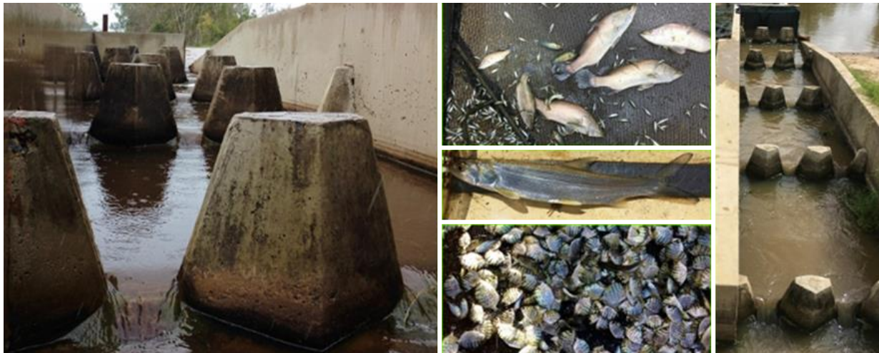
Figure 13. Concrete cone fishway on Boundary Creek, Koomala; showing fish successful at ascending, top to bottom; juvenile barramundi and empire gudgeon, giant herring & over one thousand juvenile banded scats & threadfin - silver biddy.
