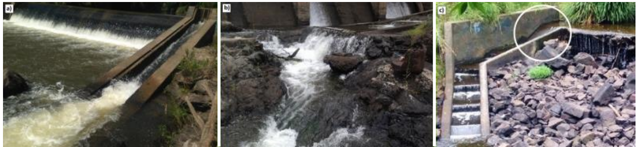
Figure 3. Showing northern hemisphere ‘salmonid’ style fishway designs exhibiting hydraulic conditions in excess of the swimming abilities of most native freshwater fish species. a) Denil fishway located on Luscombe Weir (Albert River, QLD) showing steep gradient and excessive velocities (note baffles removed). b) Showing the bottom section of the Mt Crosby weir pool and weir fishway (Brisbane River). Note the inadequate fishway entrance with excessive turbulence associated with the large water surface drop and shallow entrance pool and c) Pool and weir fishway located on the Bremer River (Berrys Weir). The exit of this style of fishway has a 600 mm high drop and velocities during base flows of 3.3 m/sec.
