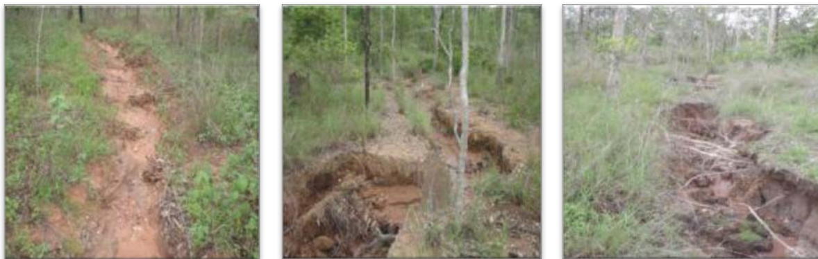
Figure 2 Examples of gullies emanating from road drains within the study area. 42% of road drains in the study area were found to have gullies like this associated within them
