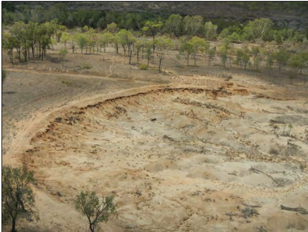
Figure 37: Example of a regraded alluvial gully in the Bowen catchment of unknown age with a constructed berm to exclude overland flow from the gully and with no soil treatment. This is the equivalent of the plot 1 control site - in which the gully is regraded with only direct rainfall driving high levels of ongoing erosion.
